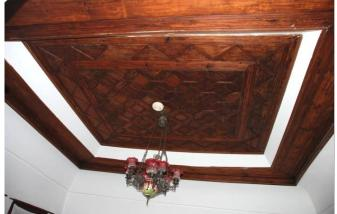
Figure 11. Lath-and-plaster workmanship of the ceiling representing Citakari artisanship and its joint with the wall - Kaymakamlar House.
