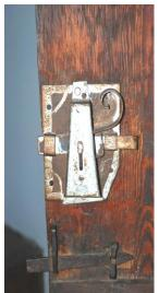
Figure 14. Use of metal material as lock and pusher on door - Kaymakamlar House.
