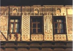
Figure 12. Application of Malakari technique on the façade of room - Mektepçiler House. [3]
