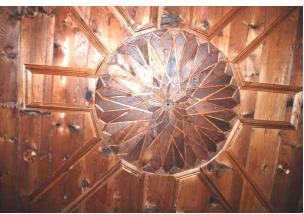
Figure 6. Ceiling and lath-and-plaster workmanship with Citakari technique - Kileciler House.
