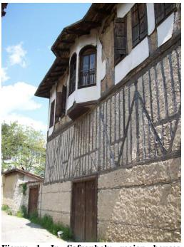
Figure 1. In Safranbolu region houses ground floor is masonry and upper floor is wood carcass. In some samples façade is coated.
